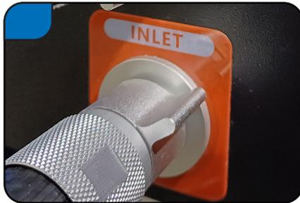
The hoses are identical and can be used on either INLET or OUTLET. Thread one end of a hose onto the INLET located on the rear of the chiller.
