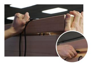
**9.** Locate the left hand bench support and slide it into place using the pre-mounted slots, making sure the heater cable is on the right hand side. Secure the right hand bench support into the left hand bench support using 2x 3\* 30mm screws & secure the right of the right hand bench support into the side wall using 2x 3\* 30mm screws.
