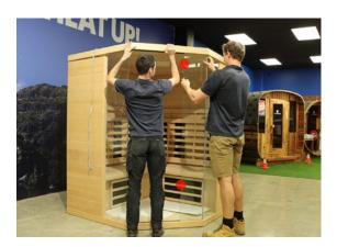
**15.** Secure the roof panel in place using the 4\* 40mm screws.
