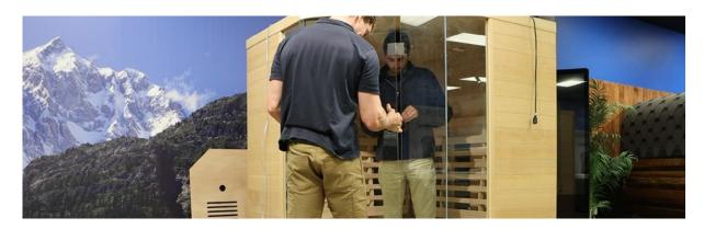
**19.** Install the magnetic seal to the door and the left hand glass panel. The magnetic seal will need rotating to match the profile below.
