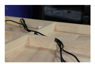
**23.** Before installing the roof covers, it's advised to plug the sauna in and check all heaters and lights are working as expected. Once you have confirmed the sauna is in working order, make sure the roof cover is oriented correctly, the vents should have cut outs above them and the controller should have breathing slots above it to prevent overheating, pull the 15A cable through the pre-cut circle hole. Secure using the 3\* 16mm screws around the outside edge.
