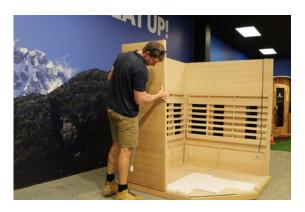
**5.** One person will need to 'rock' the left rear wall back to allow the male clasp to line up with the bottom of female clasp, once these are lined up, slowly lower the back wall down onto the side wall. You may need to gently tap the side wall towards the rear wall and/or gently tap the top of the side wall downwards to allow the clasps to lock into each other.
