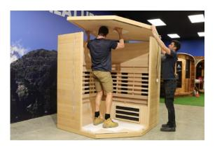
**8.** With the roof panel sitting (Not secured in place), feed all the cables through the adjacent hole in the roof panel. Once they have all been fed through, gently lower the roof into place onto the dowels, have one person go around and make sure each cable is free and not pinched between the walls and roof.
