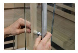
**18.** Have one person inside the sauna with the left over hinge parts and the allen key while the other aligns the door into place and lifts it so the hinge studs push into the side glass panel. Install the internal hinge through the glass with the plastic shim in place, lift the glass door as high as possible before tightening the screws all the way. Test the door and make sure that it swings freely, if it makes contact with the top or bottom, loosen off the screws and re-adjust.
