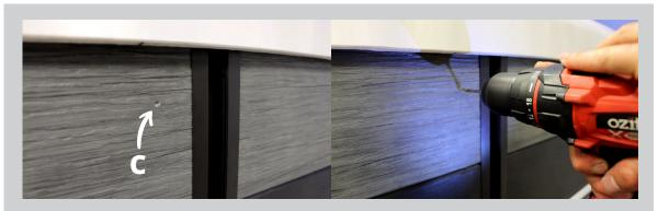
Switch to a 4mm drill bit, then drill through the cabinet panel and all the way through the steel at the guide mark (C) you made in step 4. This may take some time, be patient and apply steady pressure. Make sure the drill remains perpendicular to the spa cabinet while drilling.
