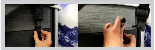
Next, with the bracket in the closed position, place the securing buckle against the swim spa cabinet. Disconnect the strap while holding the buckle in place. Use a pencil to mark the position of the buckle. This will act as a guide to assist you placing and screwing in the buckle.
