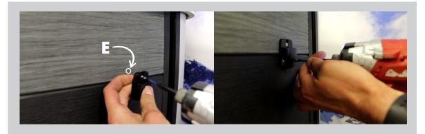
Using 3 of the six small screws provided, secure the buckle in the position you marked (E) in step 8. These screws are self-tapering so no pre-drilling is necessary.
