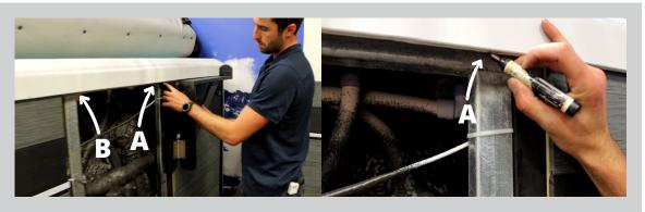
The holder will need to be screwed through the cabinet panel and into the steel frame. Mark a small line on the underside of the swim spa shell to show where the inner edge of the where steel frame lies (A). Repeat for the steel frame on the other side (B). This will act as a guide once you have replaced the panel.
