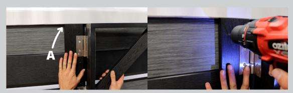
Once you have replaced the panel by reversing steps 1 & 2, place the holder bracket against the cabinet so that the hinge and cradle open outward to the edge of the swim spa. Align the inside edge of the bracket up against the mark (A) you made in step 3. Then use a 2mm drill bit to mark a guide by drilling through the top left hole of the holder (don't attempt to drill through the steel yet).
