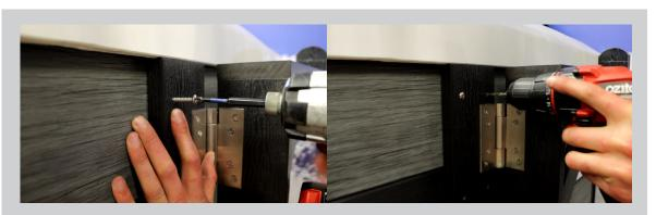
Use one of the large screws to secure the bracket in place, keeping one hand holding the bracket steady. Next, drill through the adjacent hole on the opposite side, keeping the bracket level, while applying pressure until puncturing through the aluminum vertical slat.
