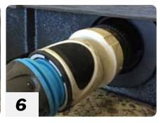
Push the drain valve slowly in towards the spa to the 'half way' point. Check that water flows from the hose and adjust (push in or pull out slightly) if necessary.
