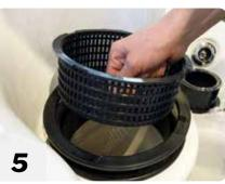
Remove the filter basket to reveal the inner weir skimmer box.
