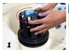
Grab the top lid with two hands, apply light downwards pressure and twist anti-clockwise to detach (can be quite stiff).
