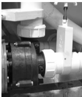
Slice Valve and Pump Union
